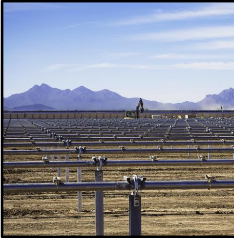
Racking Installed on posts
