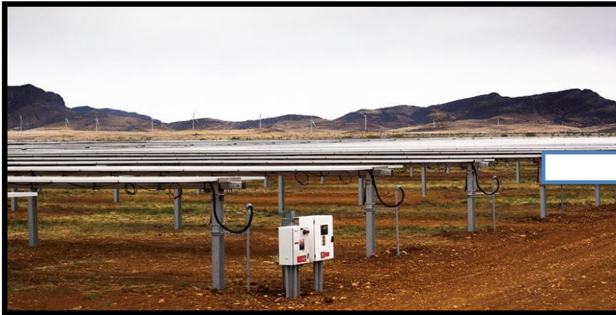
Panels Installed with Combiner Box
