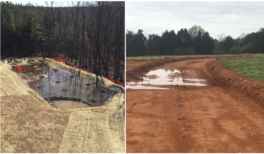
Figure 7. Example of compliance (left) and noncompliance (right) with erosion and sediment control requirements. Photos courtesy Berkley Group.
