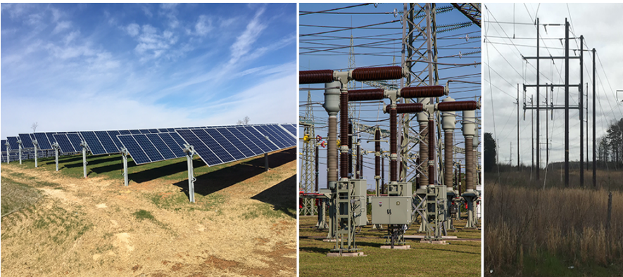
Figure 2. Components of a solar farm: solar panels (left), substation (center), and high-voltage transmission lines (right). Photos courtesy Berkley Group (left, right) and Pixabay (center).
