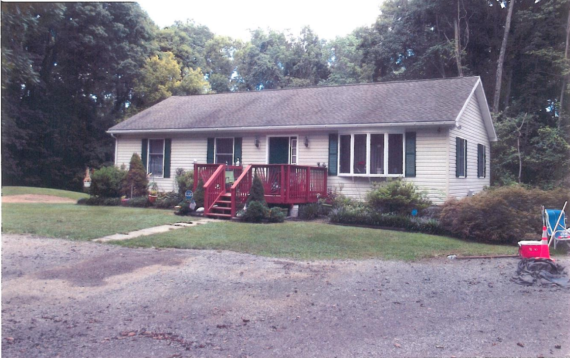
FRONT V.ew 98 FRANKLINTOWN Rd #ZV16-20
