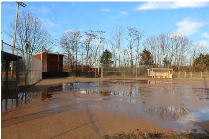
Ballfield - Note poor drainage.
