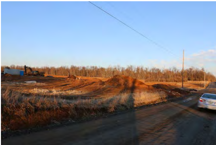
Construction progress - Spring 2015.
