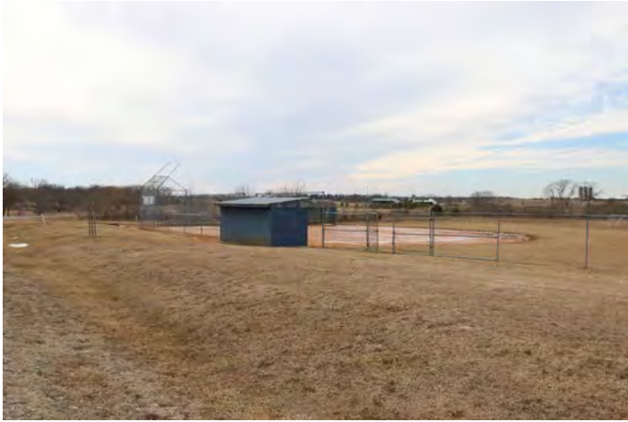
View of softball fields - Note drainage issues.
