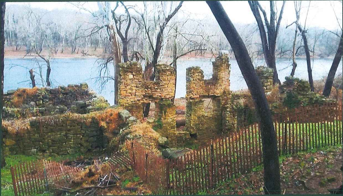
(Cement Mill building, a National Register site, Shepherdstown Battlefield)
