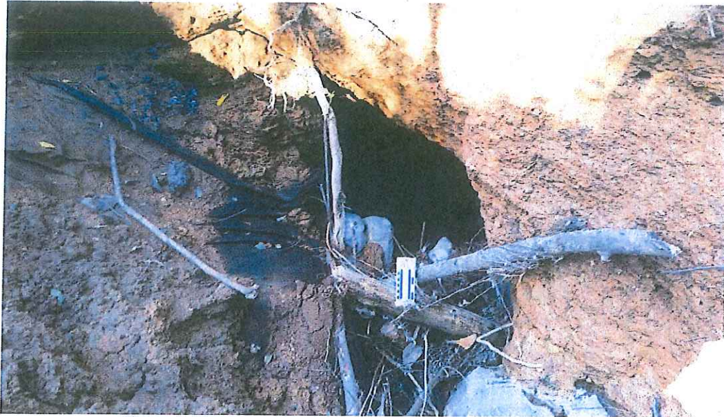
Figure 1. The cave entrance as it appeared on August 22, 2016.
