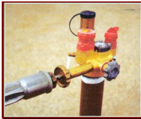
Figure 5.1.9c - Pressurizing New Vacuum Purged ASME Tank with Propane Vapor
