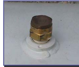
Liquid Withdrawal Valve
