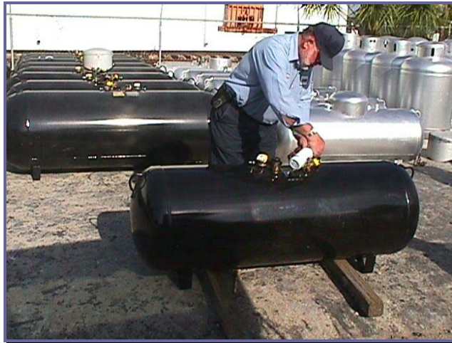
Figure 5.1.7a - Checking for Leaks on AG/UG Tank
