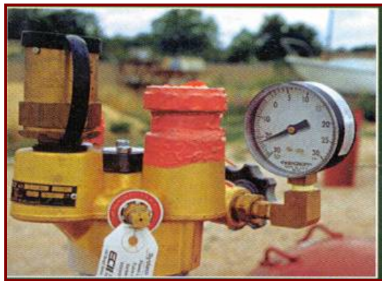
Figure 5.1.9b – New Vacuum Purged Container
