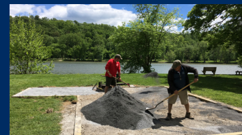
Moulton Park - Renovate and upgrade Camping Pads
