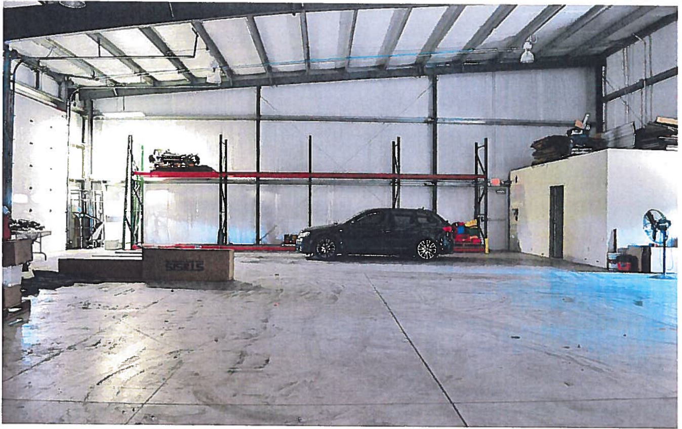
WAREHOUSE BUILDING INTERIOR
