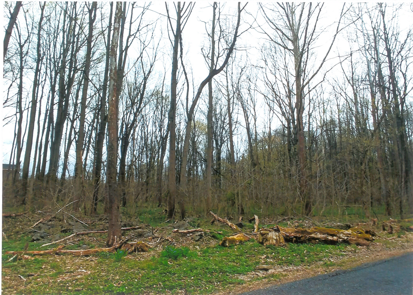
Shepherd Grade View run off / culvert area
