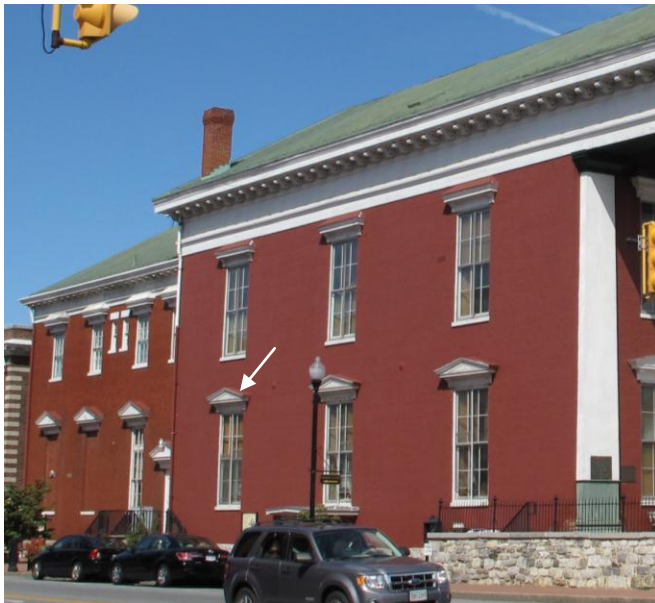
Painted Bricks and Mortar Joints on Second Story of Trapped North Elevation
