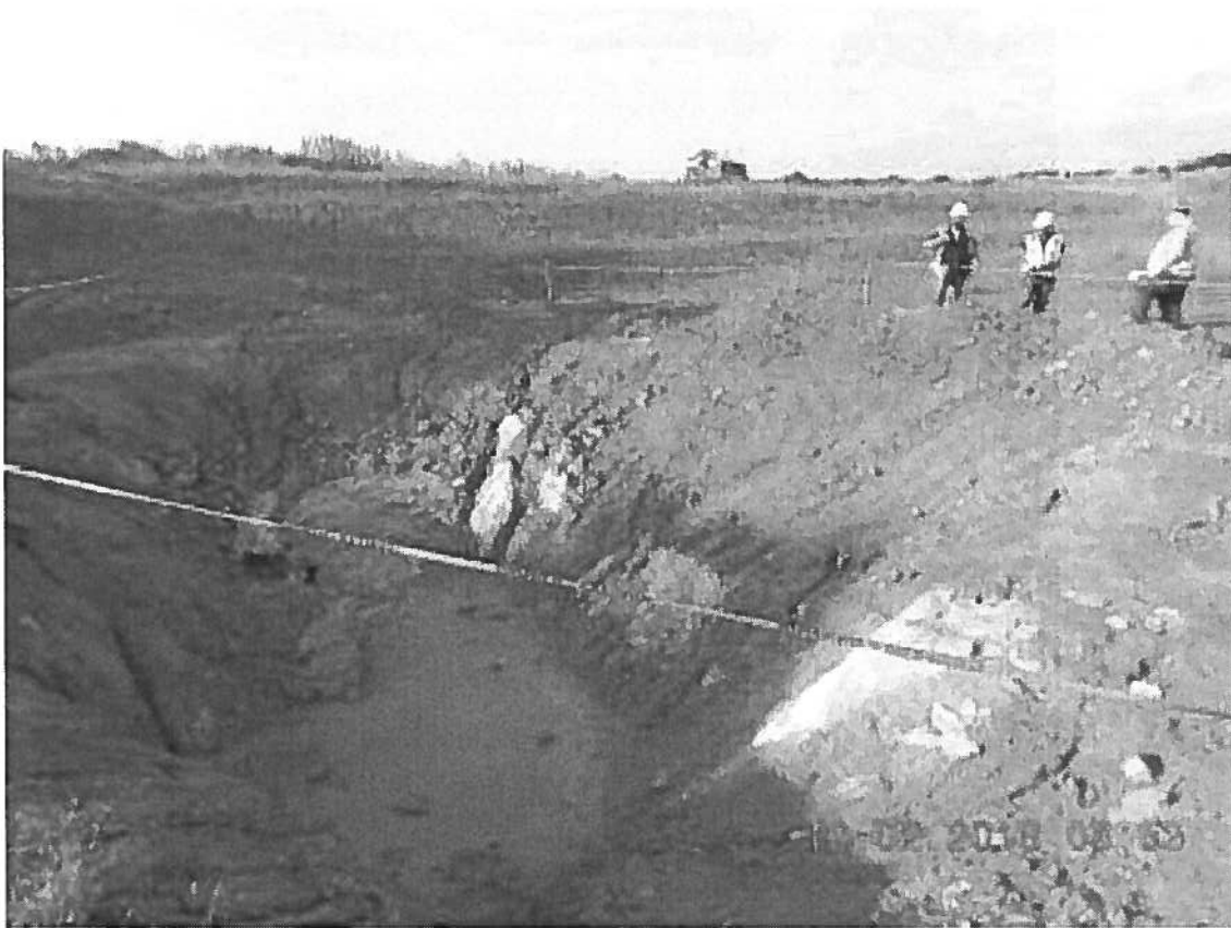
Sinkhole in Basin #1
