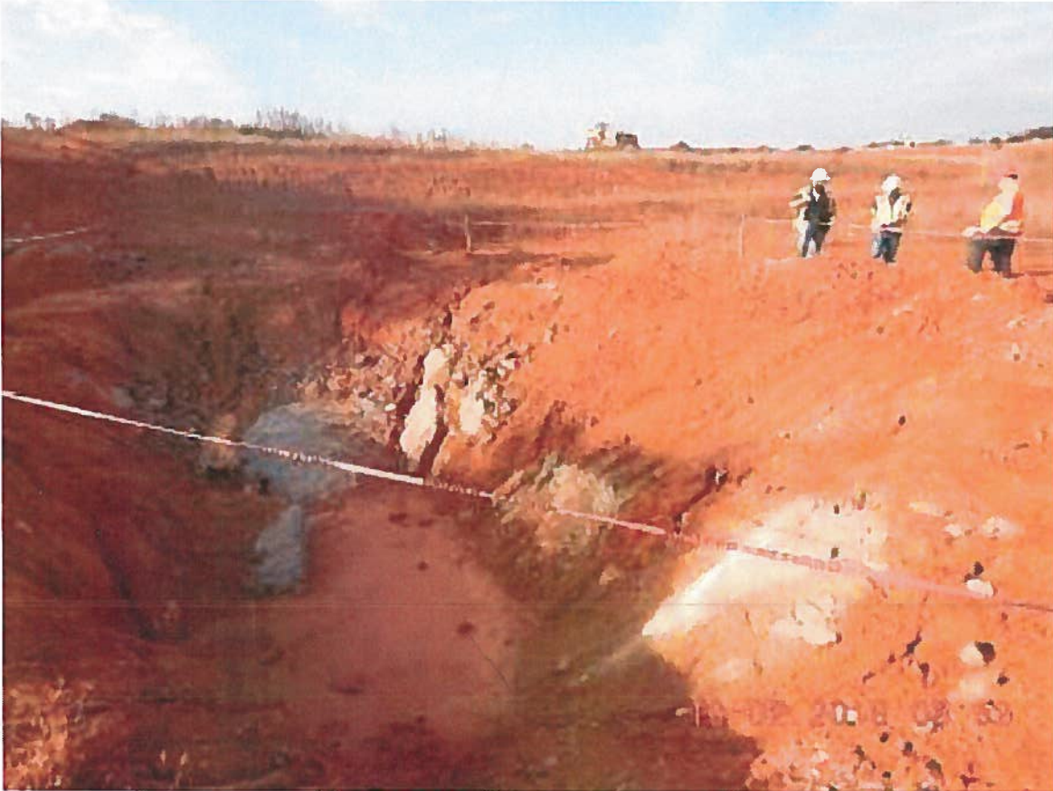
Sinkhole in Rockwool's Basin #1 – October, 2018
