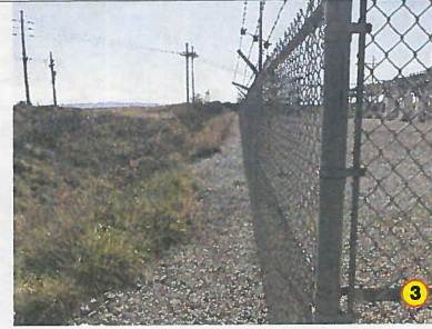
View south near balloon tether at northeast corner of substation, looking along eastern fence
