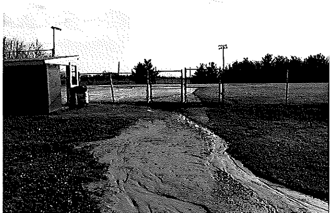
Ballfield - Note poor drainage.
