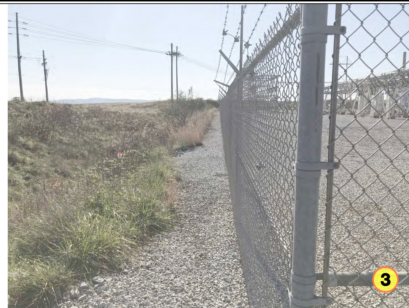
View south near balloon tether at northeast corner of substation, looking along eastern fence
