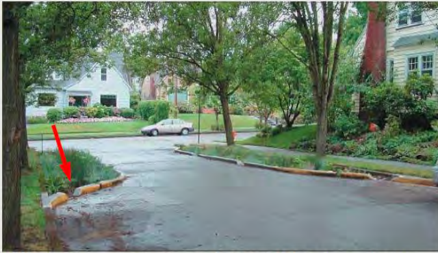
Curb Cuts permit stormwater to flow into grassy swales to reduce roadway contaminants that flow into nearby waterways. They can also be used in existing landscaped areas.
