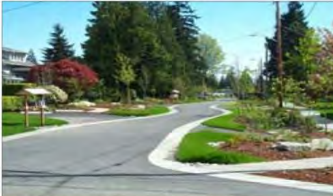
LID street design: vegetated swales, no curbs, and narrower streets promote infiltration of stormwater.
