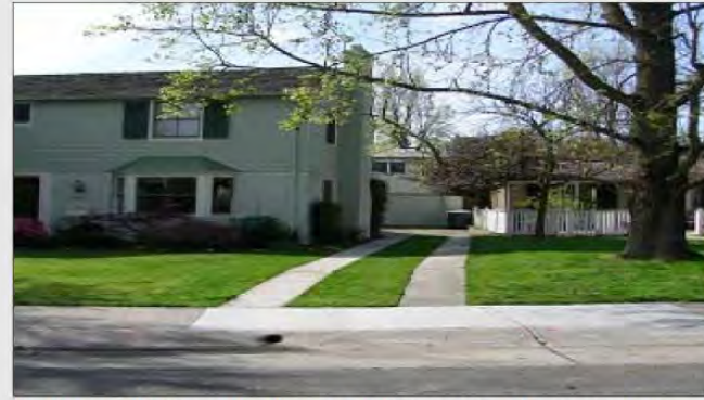
Hollywood Driveways have a dividing strip of grass in order to reduce the amount of impervious surface. Another way to reduce driveway space is to share one with a neighbor.
