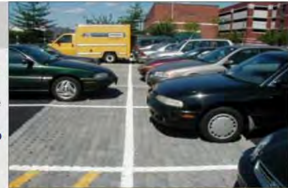
Porous pavement covers about 1/3 of each parking space in the D.C. Navy Yard parking
