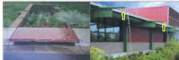
Stormdrain leading to bioretention cell
