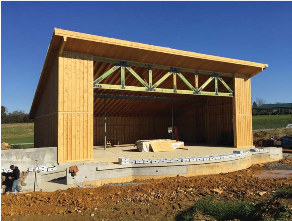
Sam Michaels Park Amphitheater Construction, October 2018
