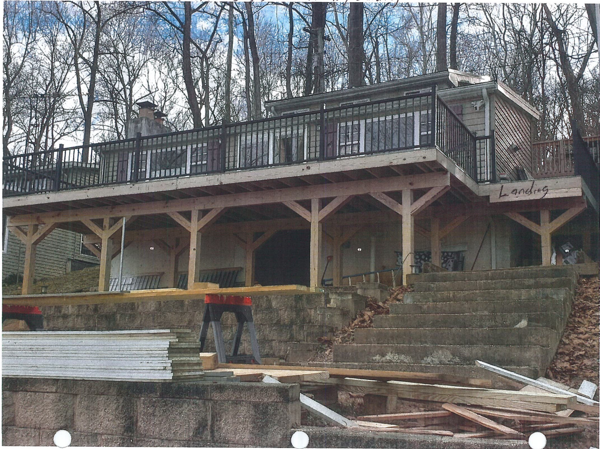
Concrete Steps Covered By Landing
