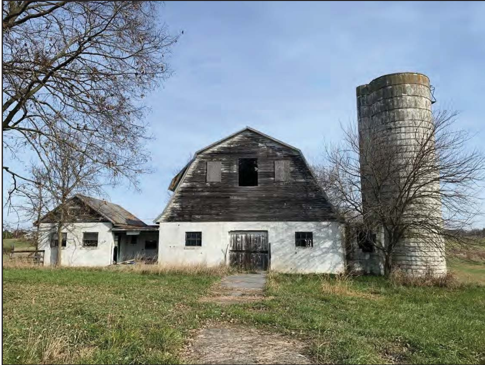
Figure 16: Barn and associate structures located on the Thorn parcel.
