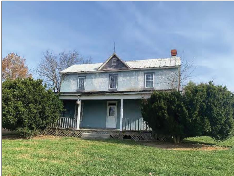
Figure 7: 1883 structure located on High Horizons parcel.
