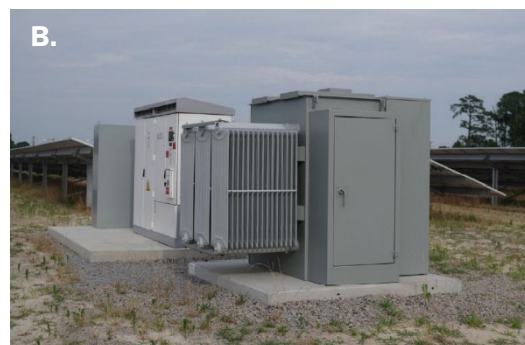
Figure 7: Inverters are installed periodically toward the interior of PV arrays.
