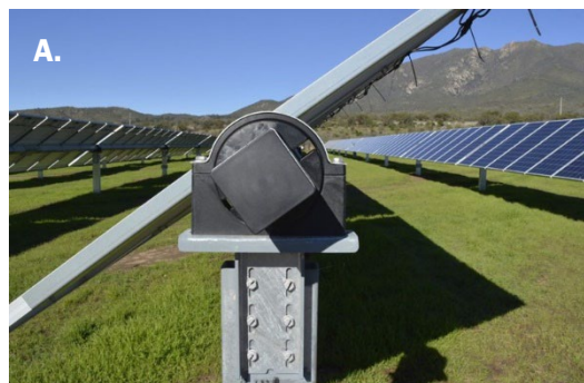
Figure 1: PV Panel mounted on Single-Axis Tracker
