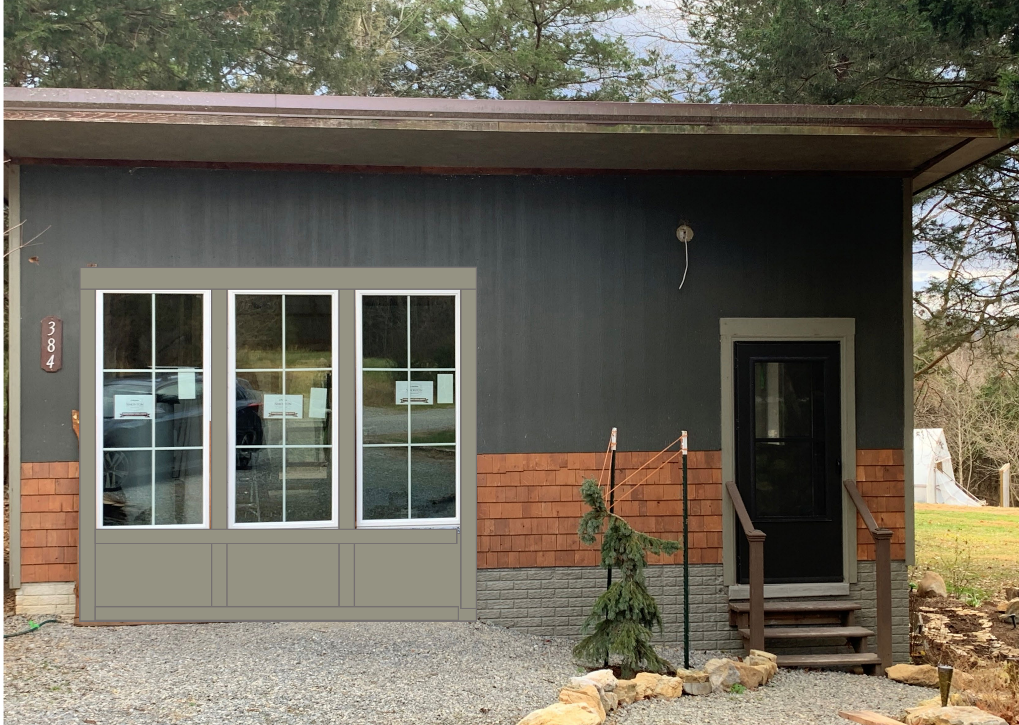
Reynes - Garage to Apartment Renovation 2022, Finished look ,visible to the road
