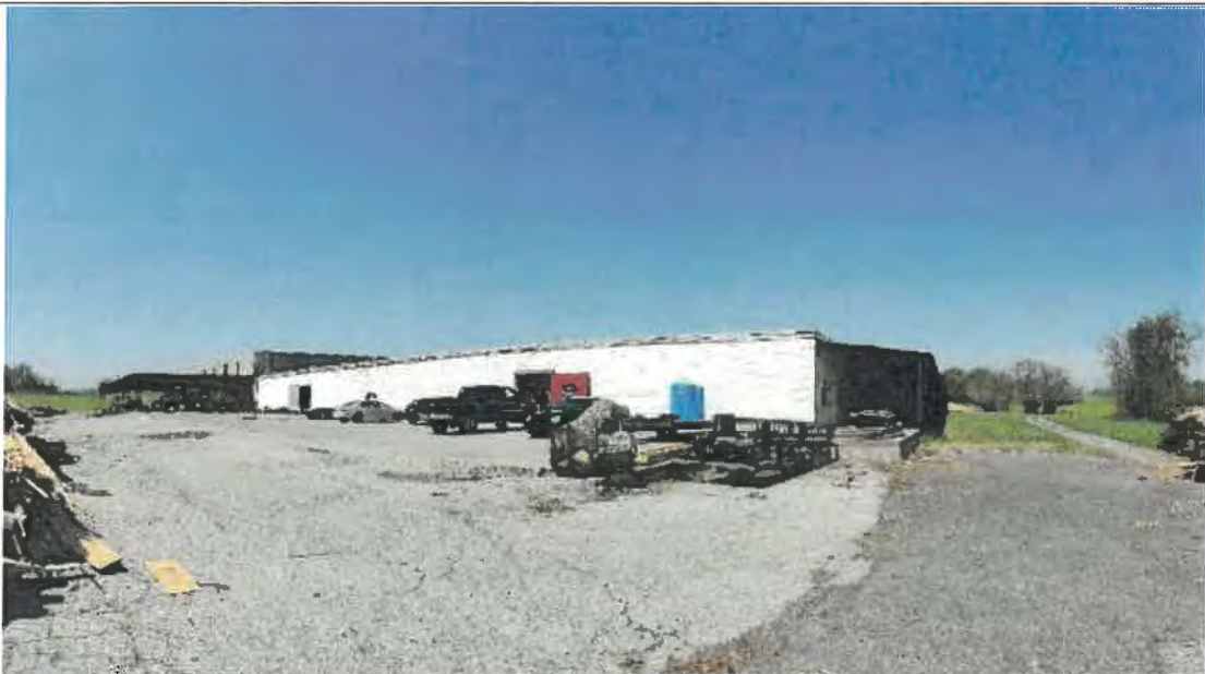
Image 8. Southwest side of the building, from the south corner.
