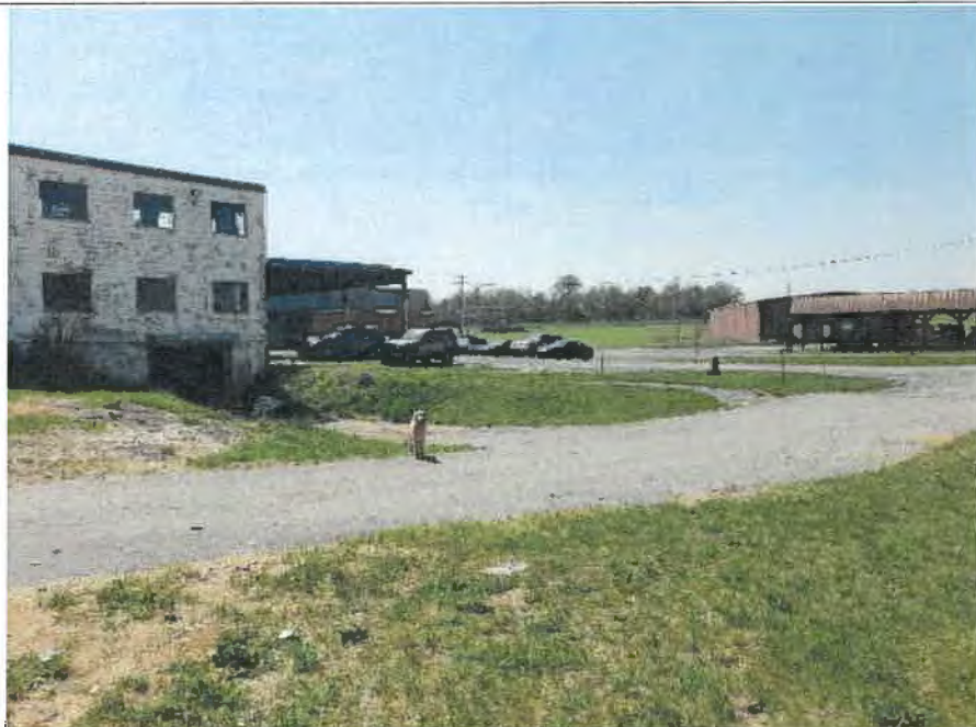
Image 12. Subject building in relation to other structures on the property. North corner of the Cold Storage building visible on the left side of the photo.
