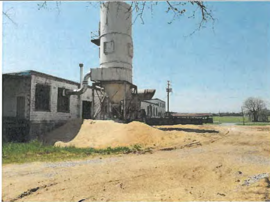
Image 11. Northeast side of the building from the east corner.
