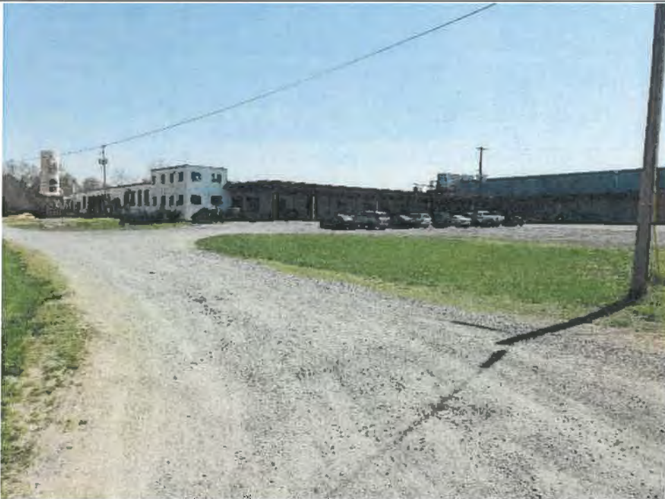
Image 4. Looking south toward the north corner of the building, with later addition visible on the right side of the photo.
