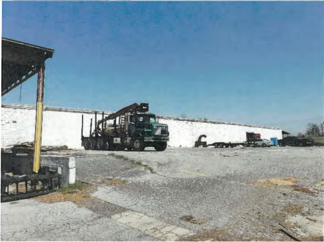
Image 7. Southwest side of the building, view toward the south corner.
