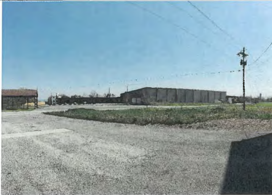
Image 5. Northwest side of the building.
