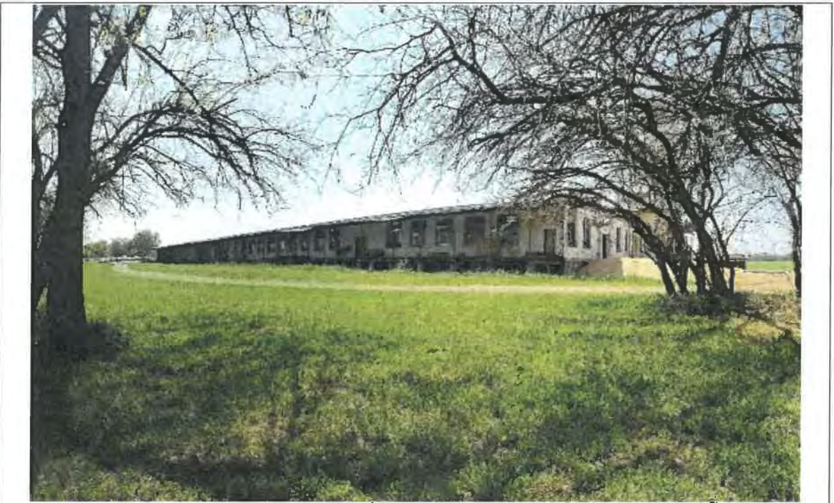
Image 10. Southeast side of the building from the east corner.
