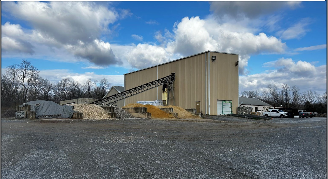
Existing concrete batch plant located on subject parcel. Applicant states this plant is used to cast concrete pavers and other concrete products.
