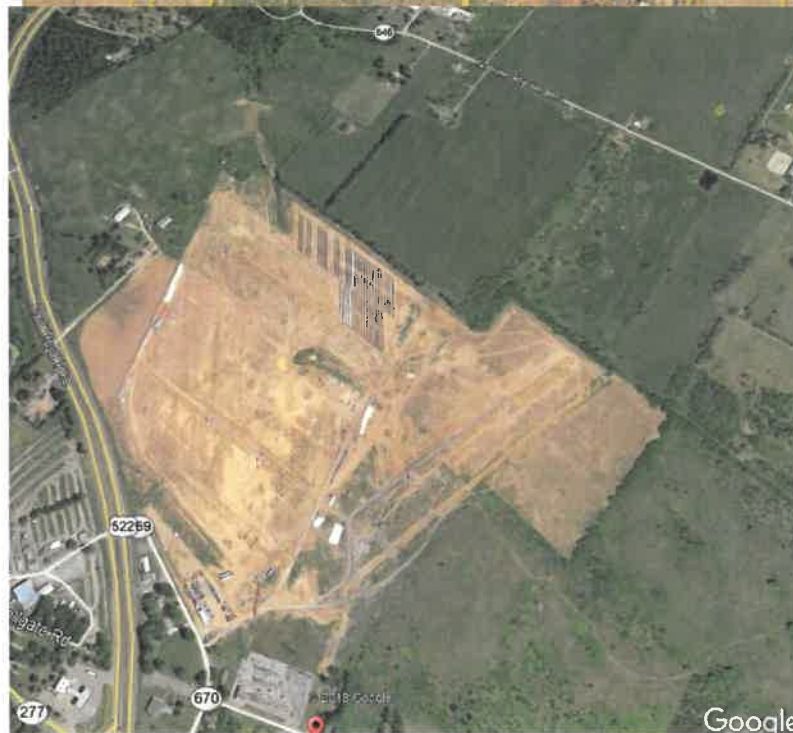
This project is a 20 MW facility located on a 234-acre tract that was built in 2017.
