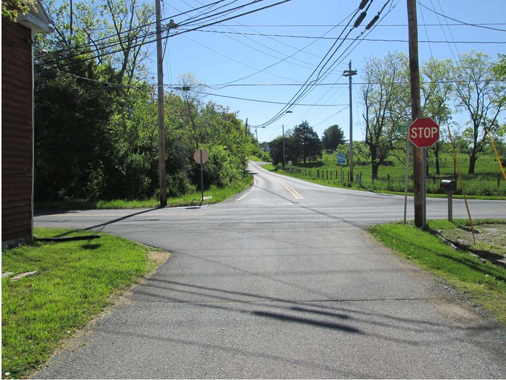
Charles Street Eastbound Approach to CR 1
