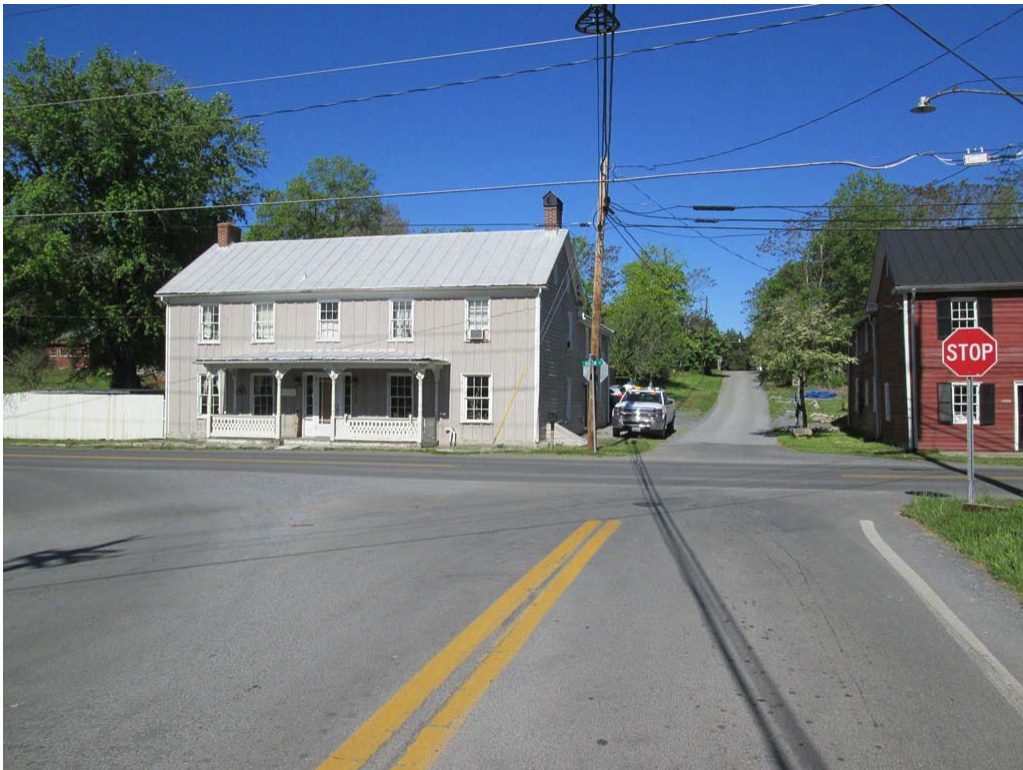
CR 1/7 Westbound Approach to CR 1
