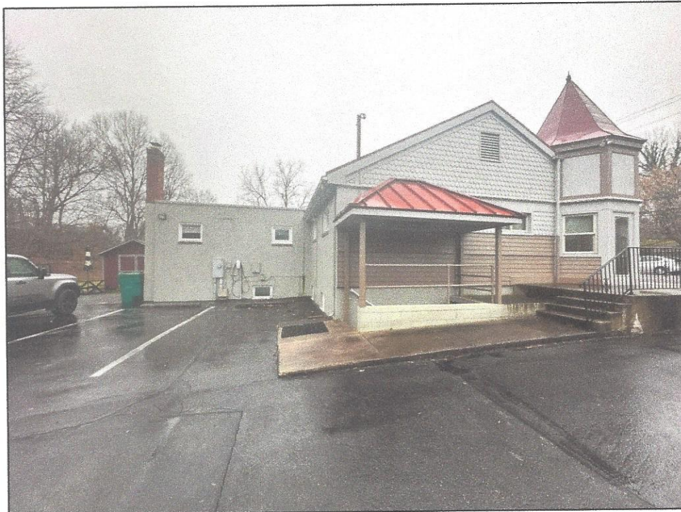
BUILDING NORTH EXTERIOR
