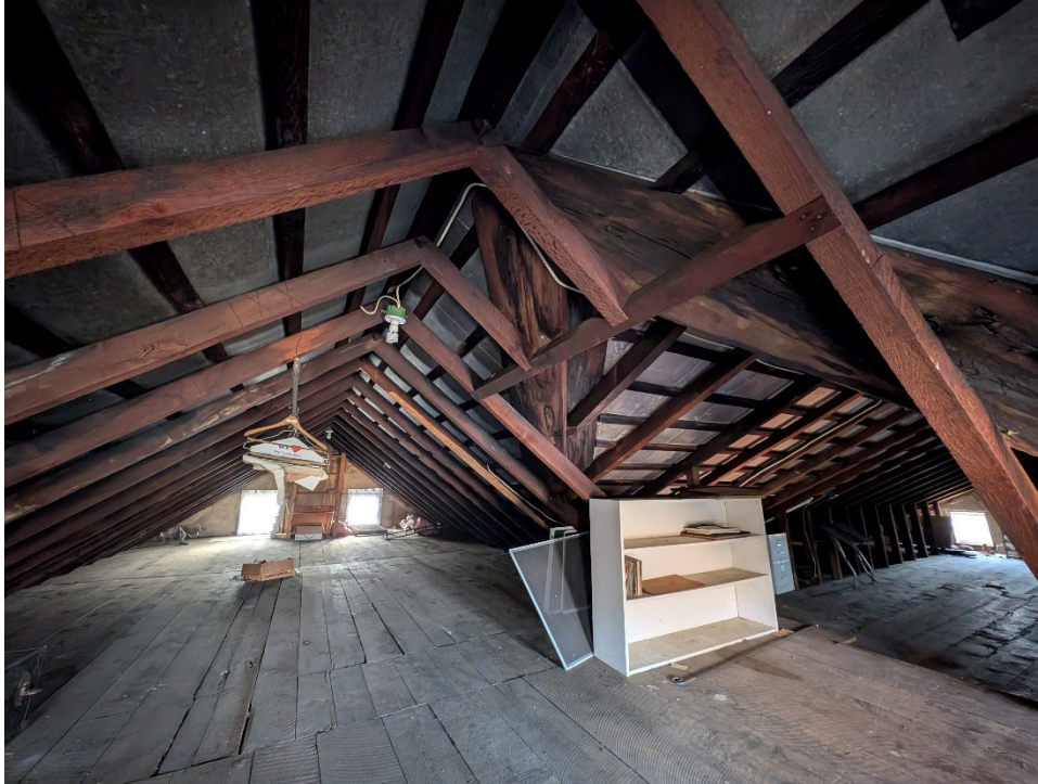
27 of 36: Attic facing southwest
