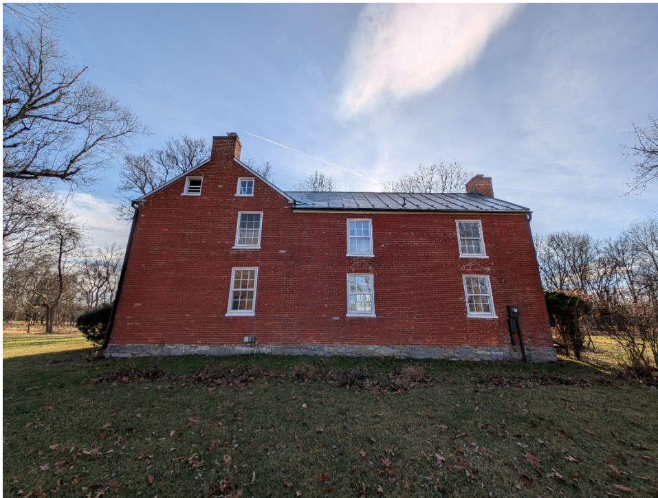
4 of 36: North exterior wall facing south
