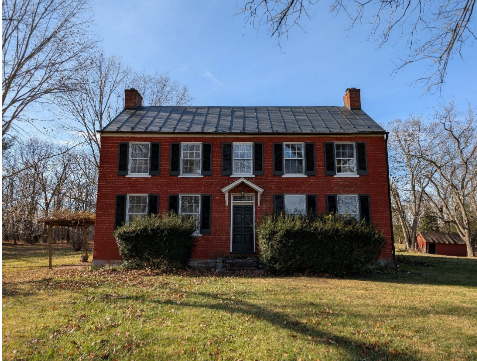
1 of 36: Façade facing west (the rear outbuilding is no longer extant)
