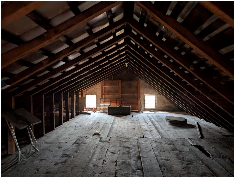
28 of 36: Attic facing west
