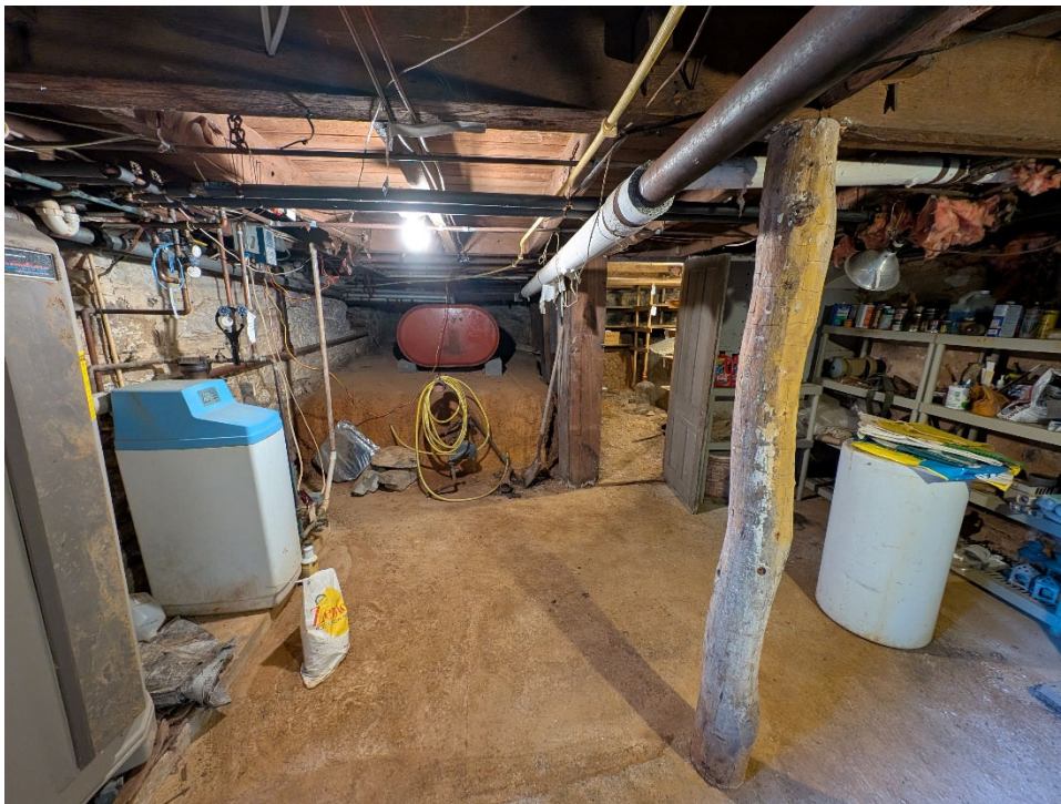
30 of 36: Basement facing north
