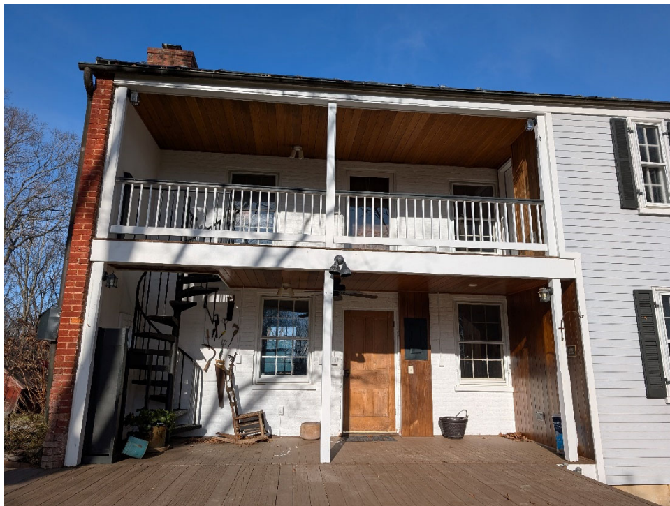
8 of 36: Rear porch facing north
