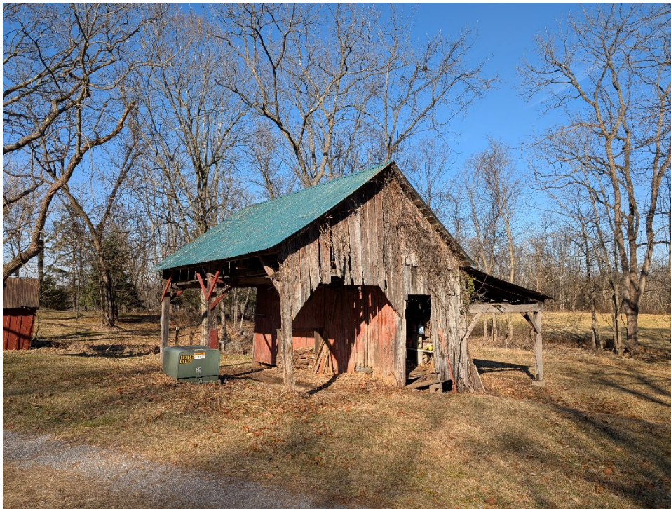
32 of 36: Corn crib facing northwest
