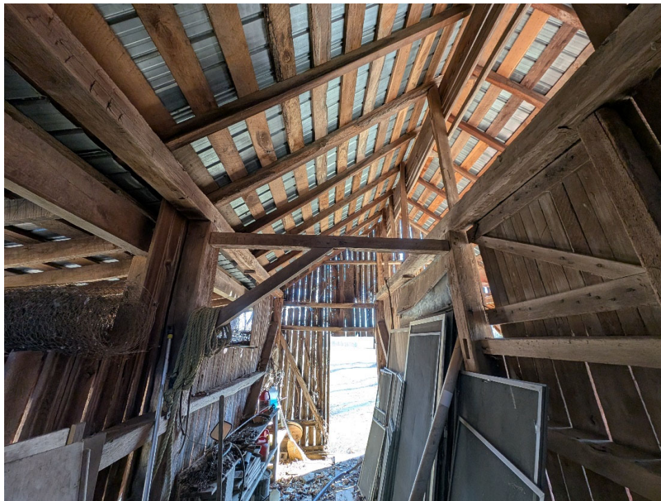
36 of 36: Corn crib interior facing east
