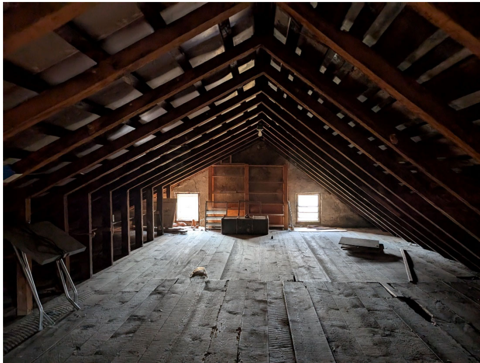
28 of 36: Attic facing west
