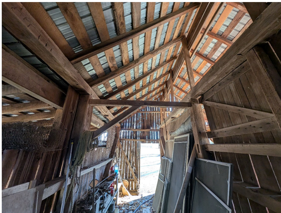
36 of 36: Corn crib interior facing east
