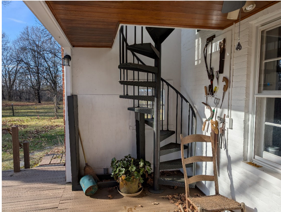
9 of 36: Spiral staircase on porch facing west
