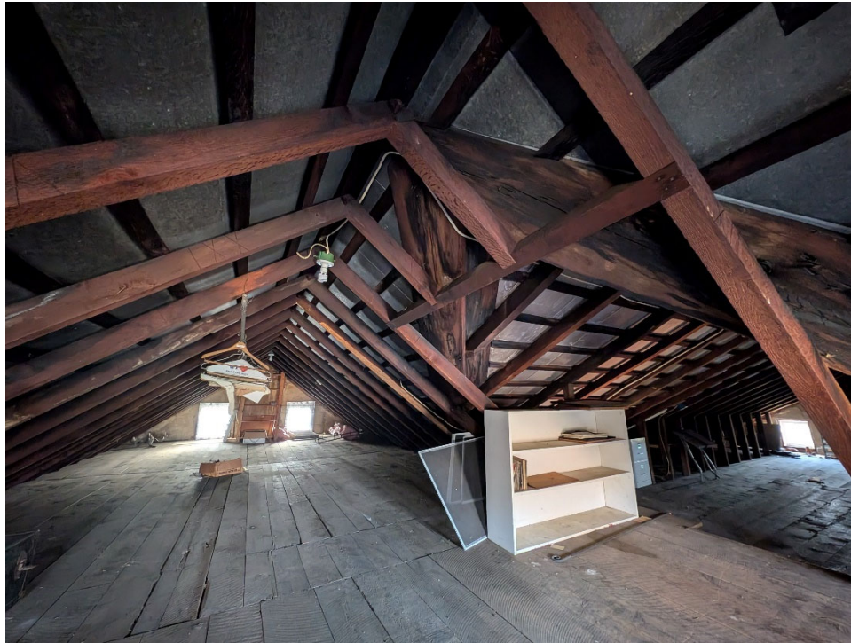
27 of 36: Attic facing southwest
