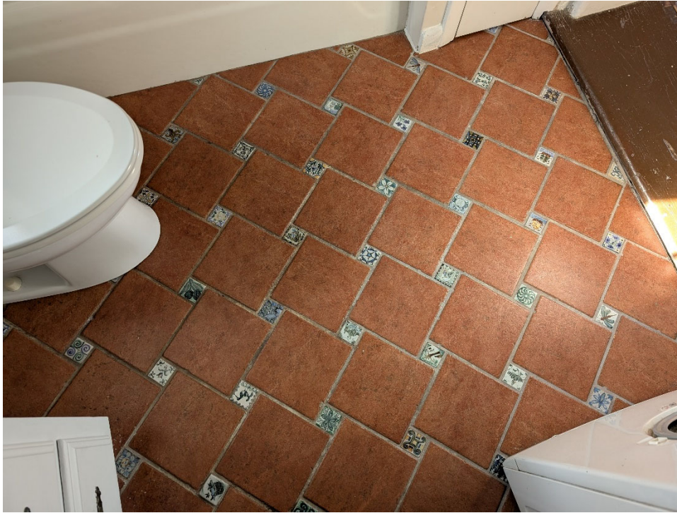
21 of 36: Detail of first story bathroom floor with non-historic homemade tiles
