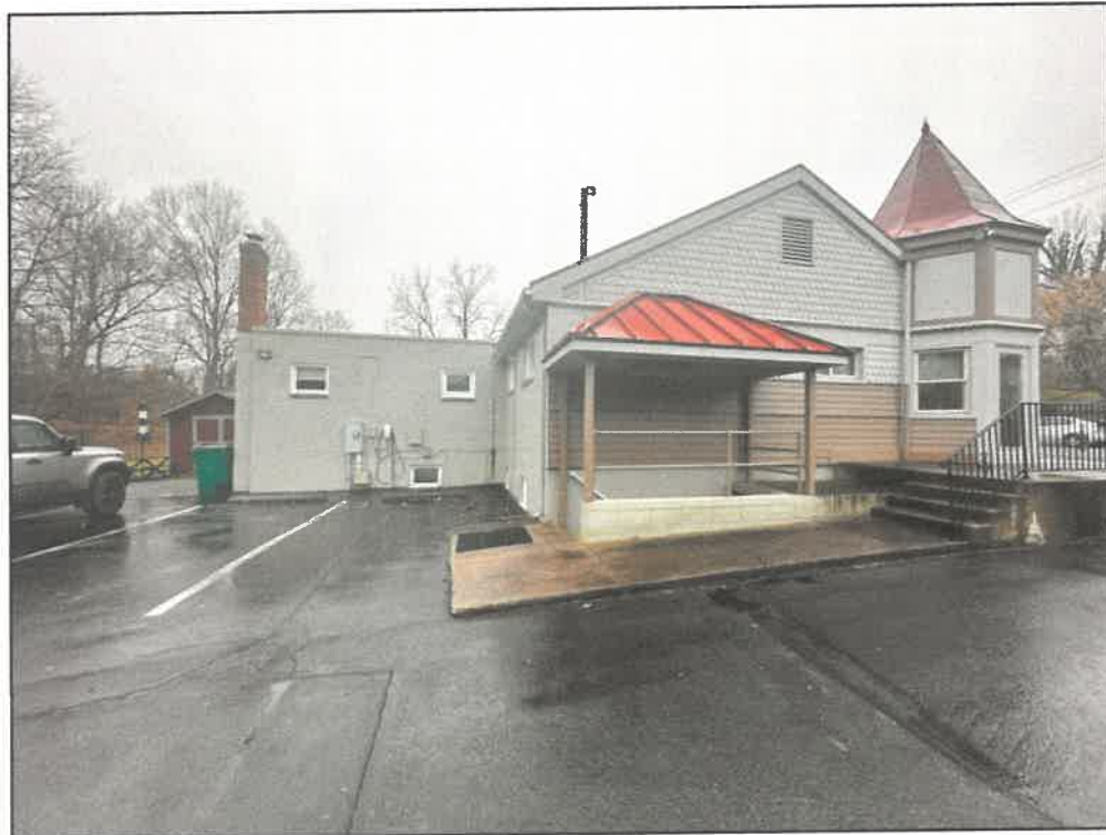
BUILDING NORTH EXTERIOR
