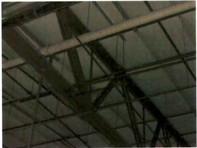
#14 Insulation on sprinkler system water pipes
