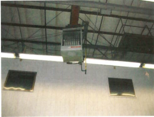
#13 Overhead propane gas heaters and insulated roof
