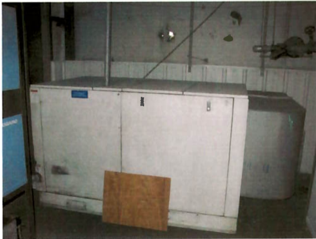
#20 One of two emergency gas fired generators
