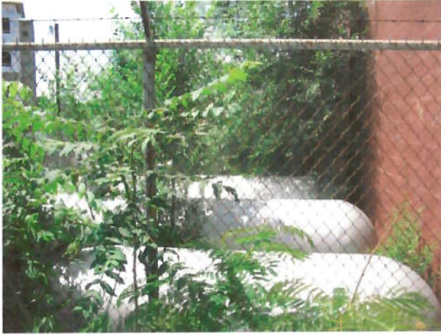
#19 Propane storage tanks in fenced enclosure with fire wall
