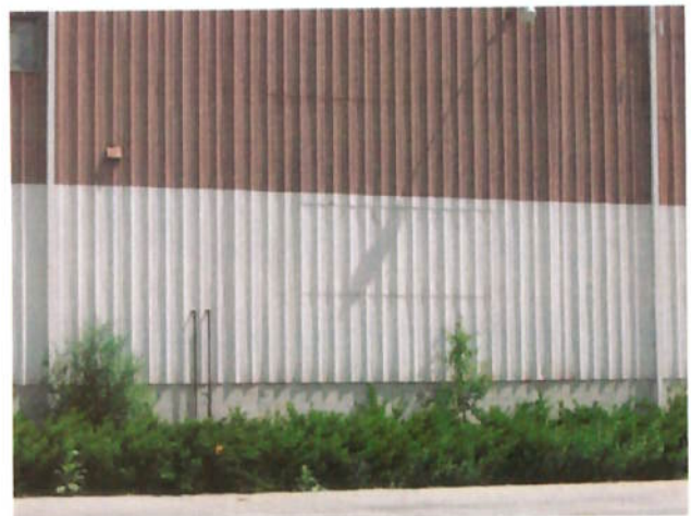
#4 South front of building, with roof rain leaders discharging to parking lot
