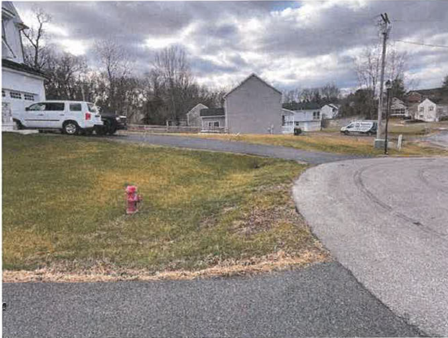
Photo taken from driveway serving Lot 3 looking south to Lot 2. A driveway culvert is present under the driveway serving Lot 2.
