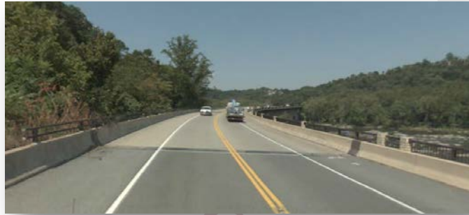
Figure 1433: Harpers Ferry Bridge at Shenandoah River, Source: Google Maps
