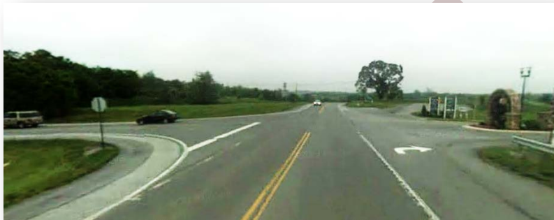
Flowing Springs Road / WV 9 Ramp
