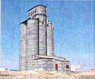
Former sugar silos now hold phone gear.
