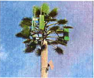
The fruit of the palm: antenna panels.
