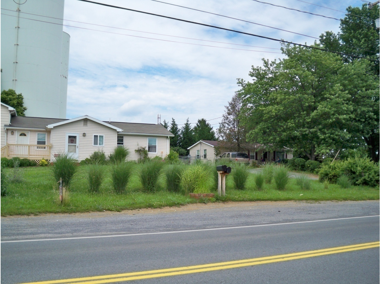
Photo 3 – Residential use to the east of subject property
