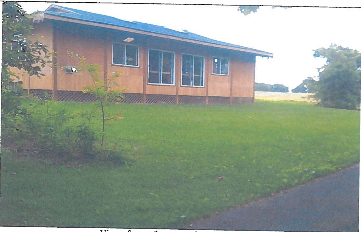
View of rear of structure from right of way
