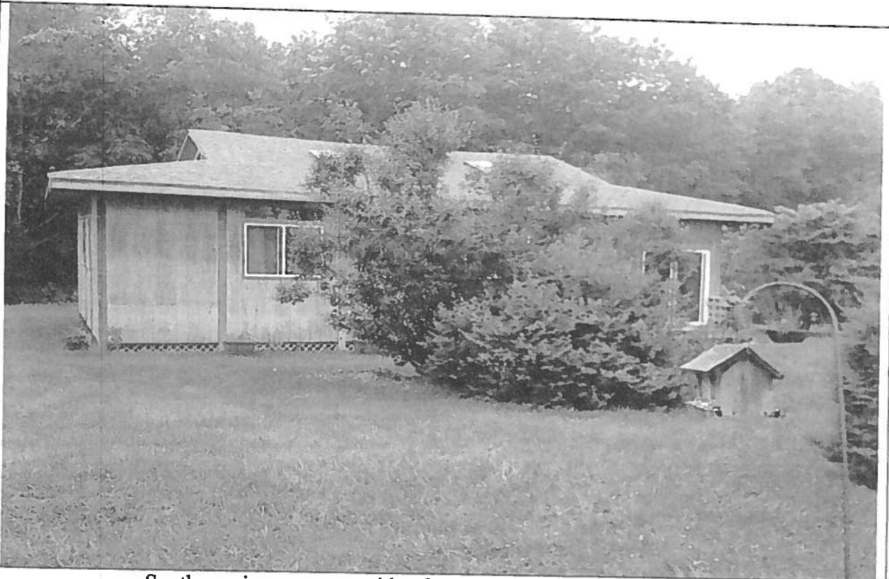
Southern view, entrance side of structure (side nearest our house)
