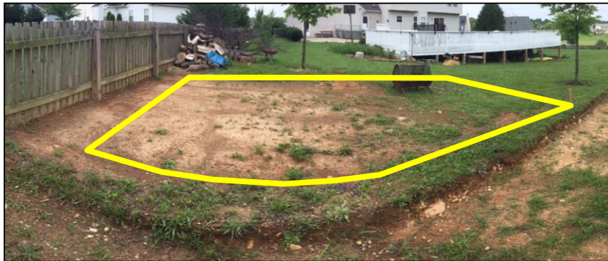
(Site location in backyard for shed; Boundaries skewed due to panoramic photo, )
