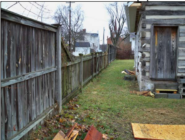
Photo along front of existing log structure facing Grace Street (to the left)
