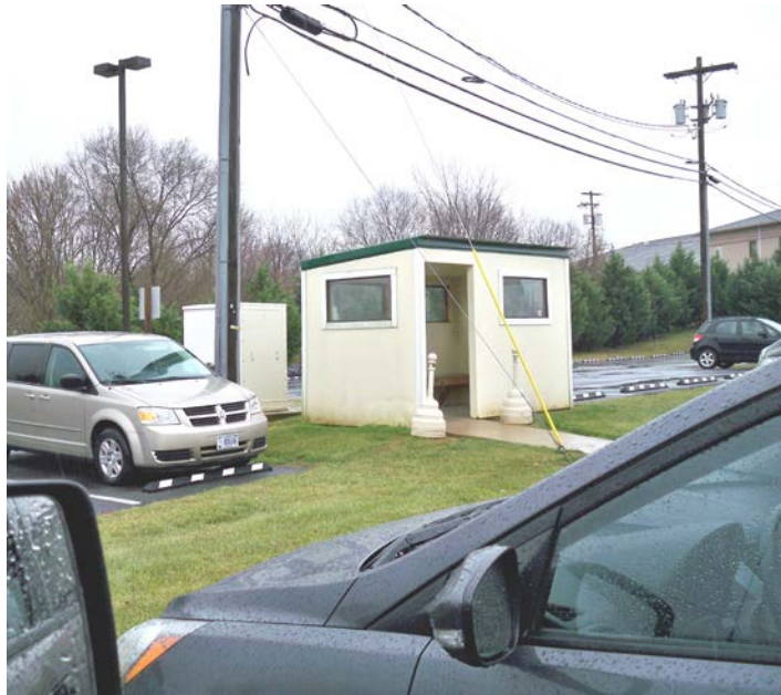
Front of Smoking Shelter located where Property line is Proposed
