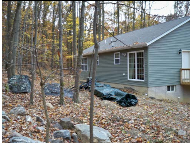
View of Rear Entry
