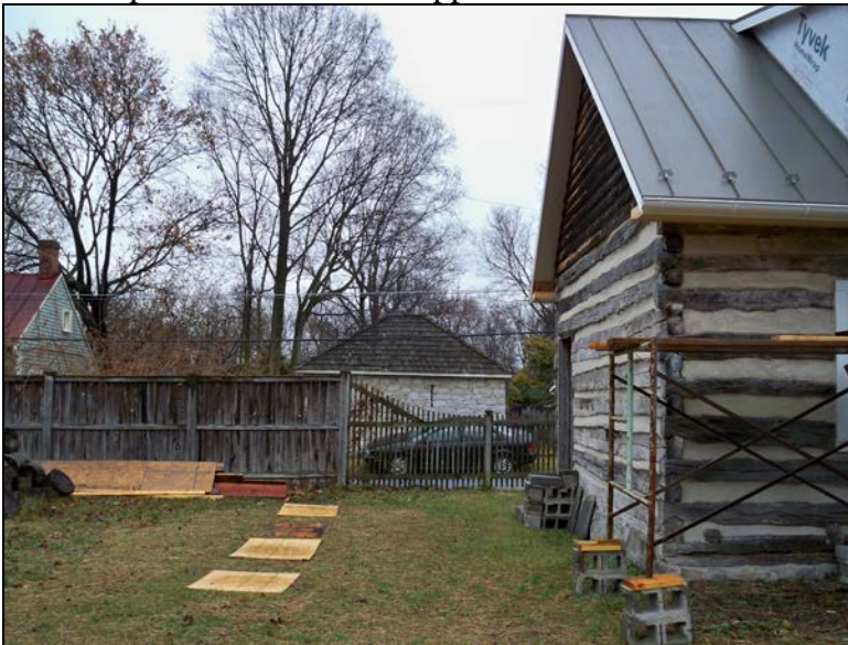
Photo of area where lean to/shed roof structure is proposed
