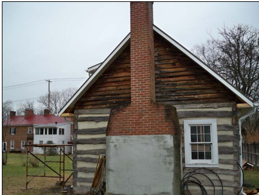
Eastern Edge of the Log Structure
