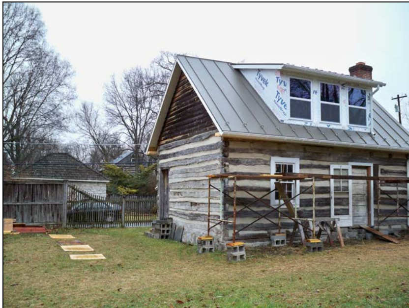
View of the Structure from inside the yard behind Scollay Hall
