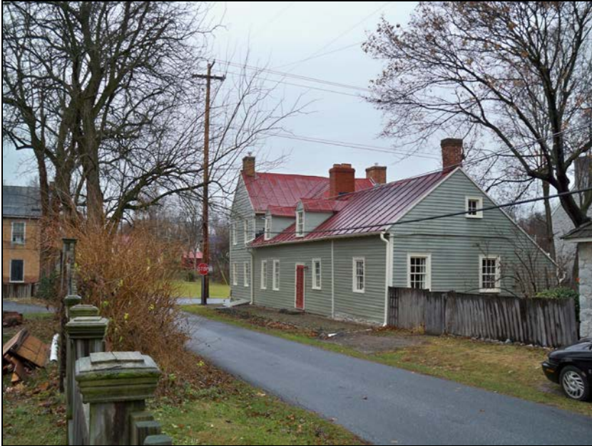
Taken from the front of the existing log structure, looking across Grace Street
