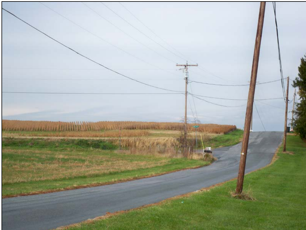
View of Ward Clipp Rd & Kabletown Rd
