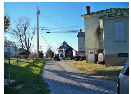
View of built section of right-of-way, facing west
