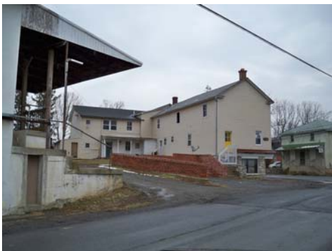
View of main house from Withers Larue Road.
