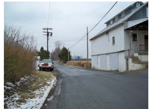
View of mill building from Withers Larue Road.
