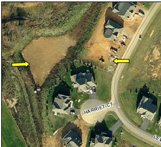
*Depicting Lot 27 and the stormwater management facility.
