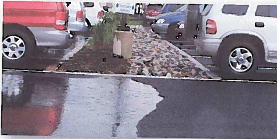
Figure 9: Examples of standard pavement alongside pervious pavement
