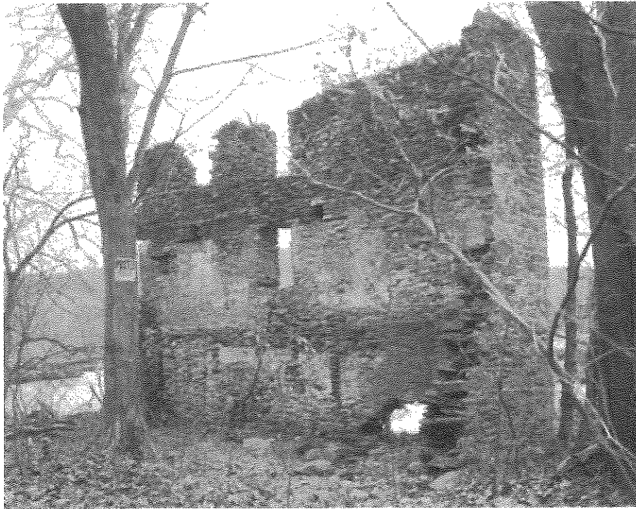
View of east interior wall with Shenandoah River beyond
