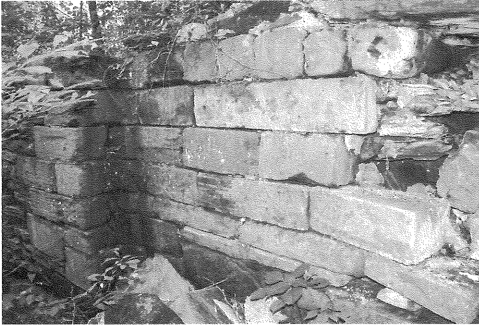
Cut sandstone lock wall – view upstream toward canal
