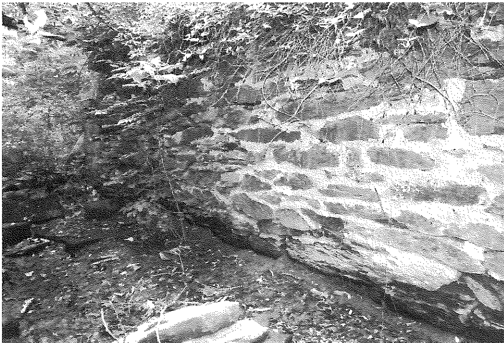
Rubble canal wall – view downstream toward Shenandoah River
