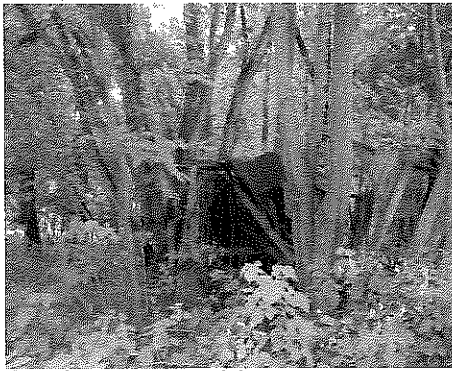
Ruined structures in wooded area
