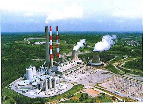
Harrison Power Station is located on 110 acres of a 1,400-acre site in Haywood, West Virginia, along the West Fork River.
