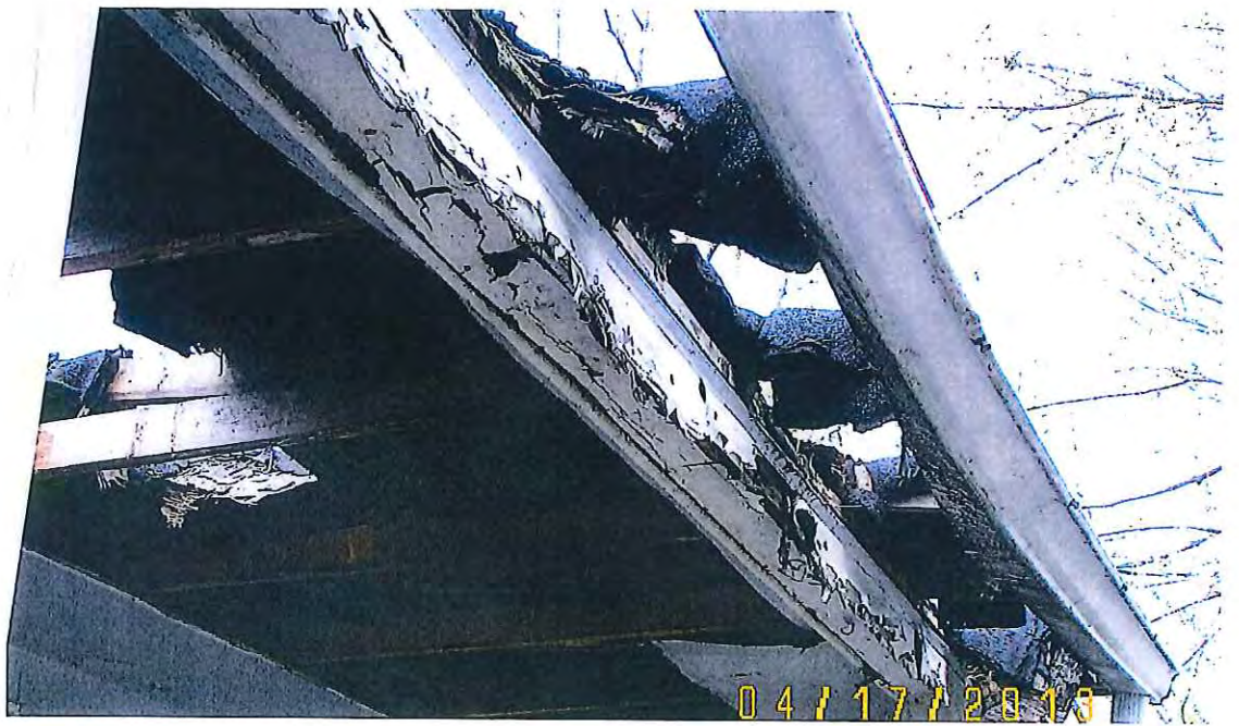
Front Porch Roof
