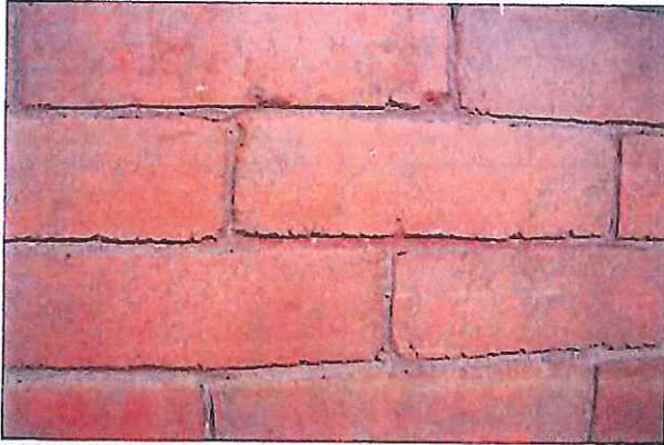
5.1.e Detail of brick in addition. Note tinted mortar.
