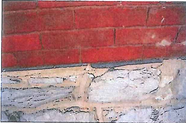
5.1.g Detail of brick and stone foundation in addition.
