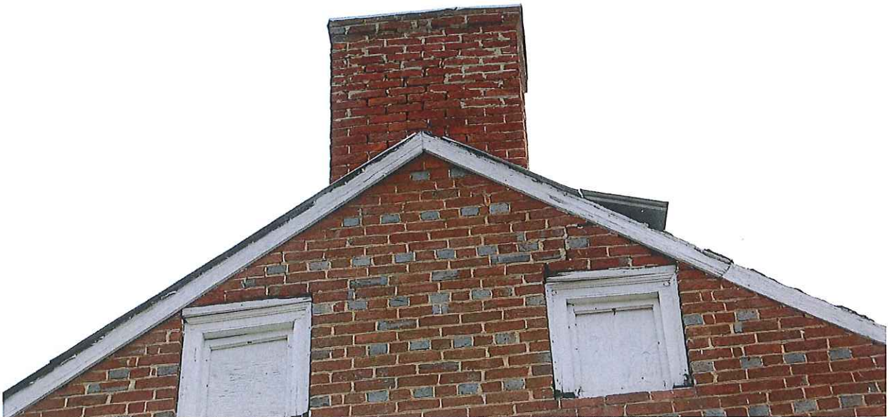
Photo #4: West side chimney detail
