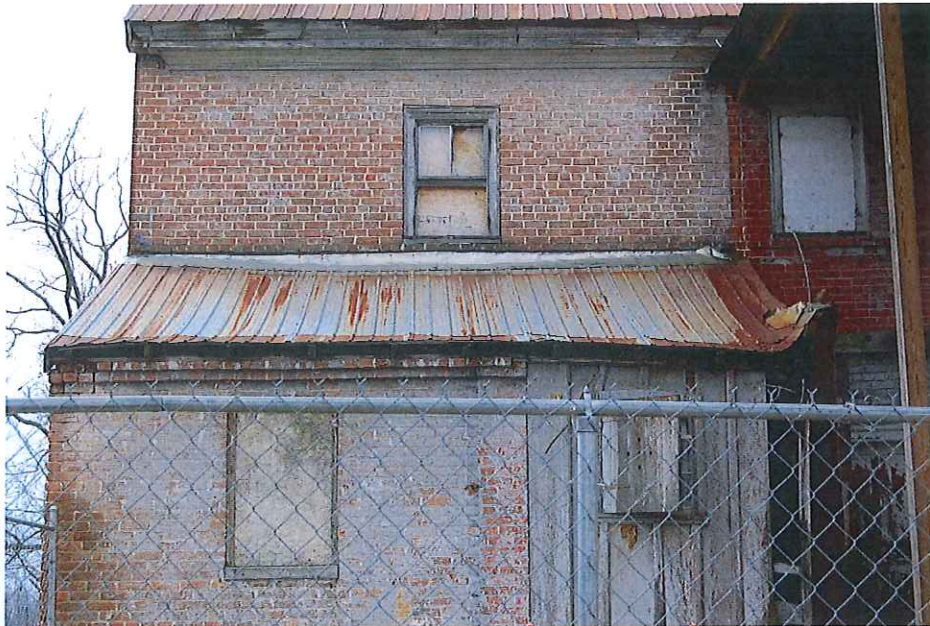
Photo #1: Addition roof, north side
